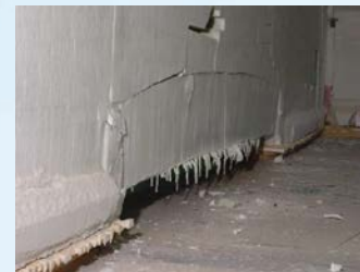
Curtain Wall of a float furnace
