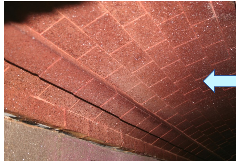
Identical furnace showing unreacted spinel crown after 6 years
