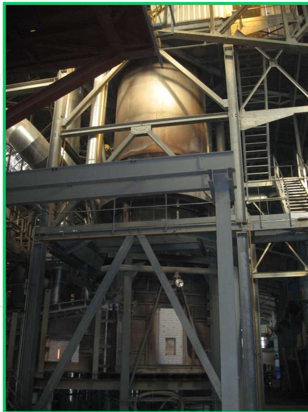
Fig. 12. Air fumes recuperators (Left) Picture (Right) Schematic view with piping and connection with secondary exchangers
